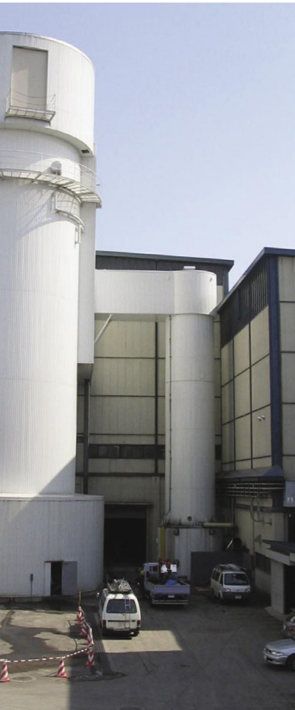
BMA extraction tower and the new pulp press HP 3000 M
